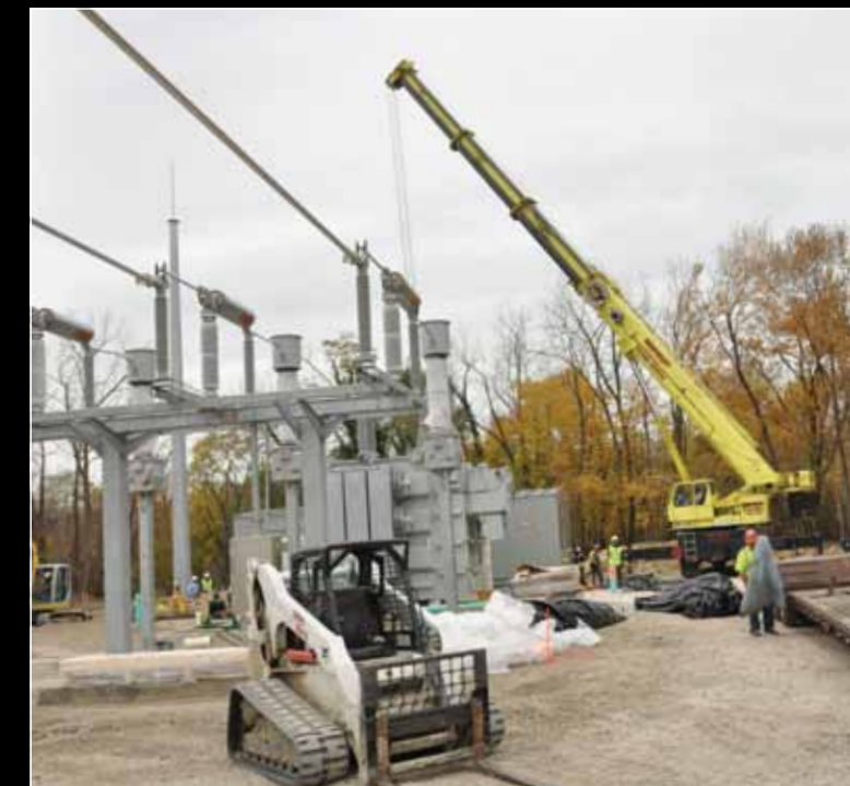
Construction is underway for the Northeast Ohio Regional Sewer District substation.
